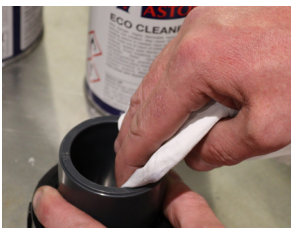
Clean pipe first
