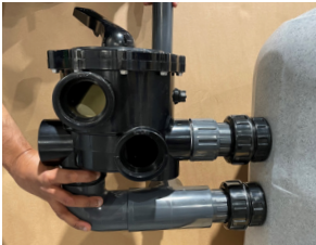
“Dry fit” pipework first
