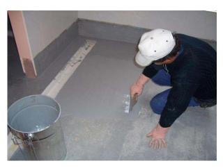
Once the first layer (primer) is cured, apply the main waterproofing layer of approx.  $1.5-2~\text{Kg/m}^2$ , mixing with SUPER ACCELERANT (1,5 L / 25 Kg of IMPERMAX). Spread the product with a toothed spreader of approx. 3.2 mm in height, and width 28 cm. The toothed spikes in the blade must be triangular, to minimise marks on the surface, and to assist in the self-levelling of the product. The product must be spread gently to avoiding the creation of bubbles.
